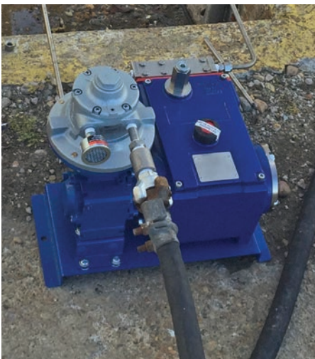
MT8 pump used for anti-scalant.
